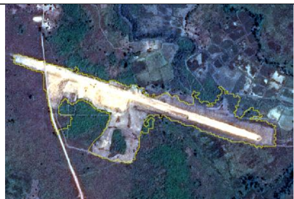
Image SPOT6 1,5m, (CN) 2015, Construction d'une route. Guinée maritime.
